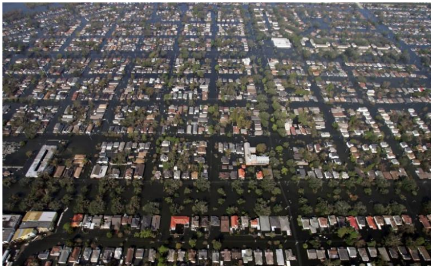
Houses remain surrounded by floodwaters from Hurricane Katrina in New Orleans, Louisiana September 4, 2005. REUTERS/David J. Phillip/Pool
